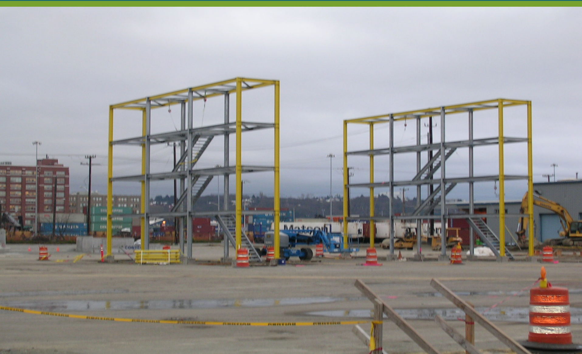
Reefer Racks Installation
