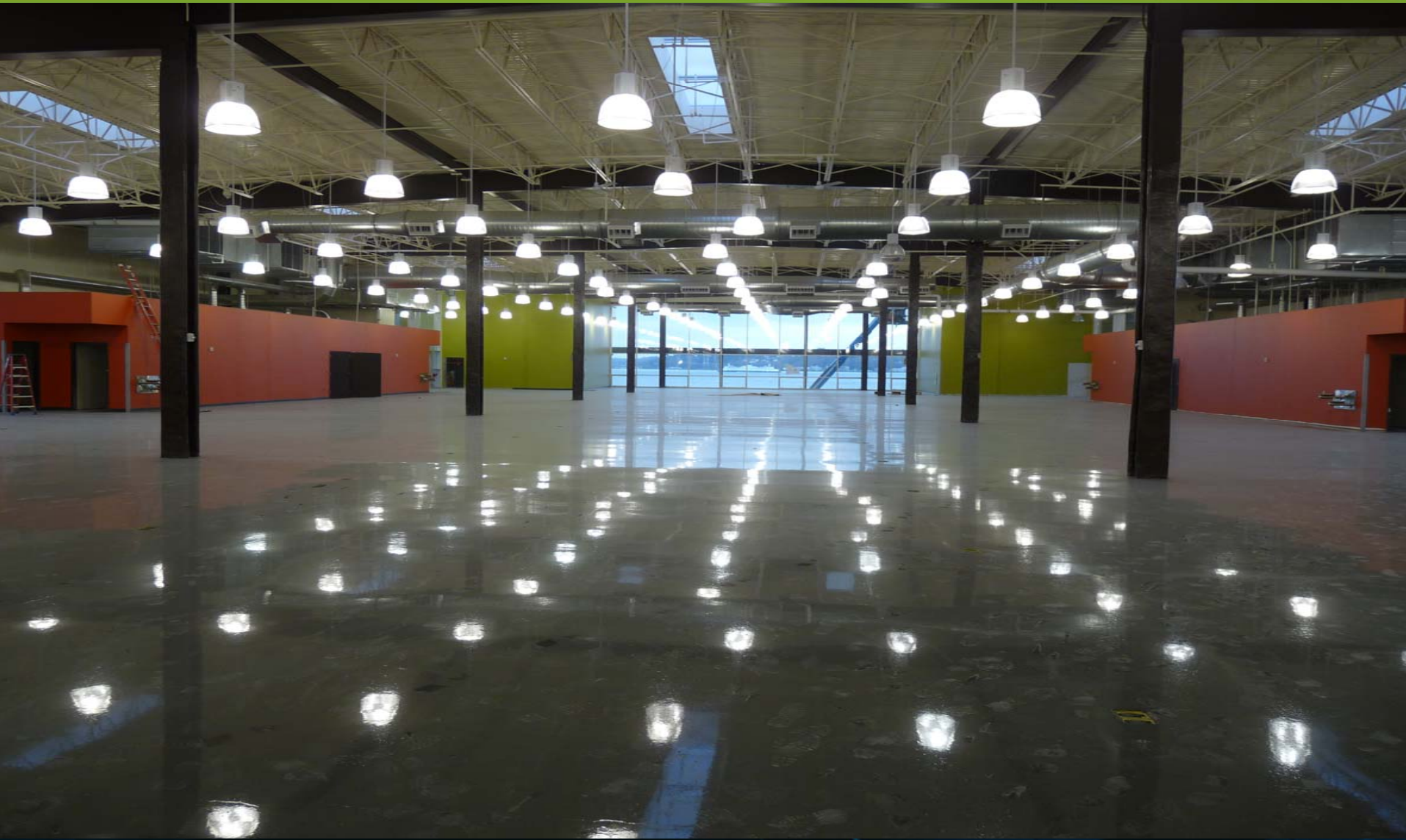
Second Level (Looking South)
