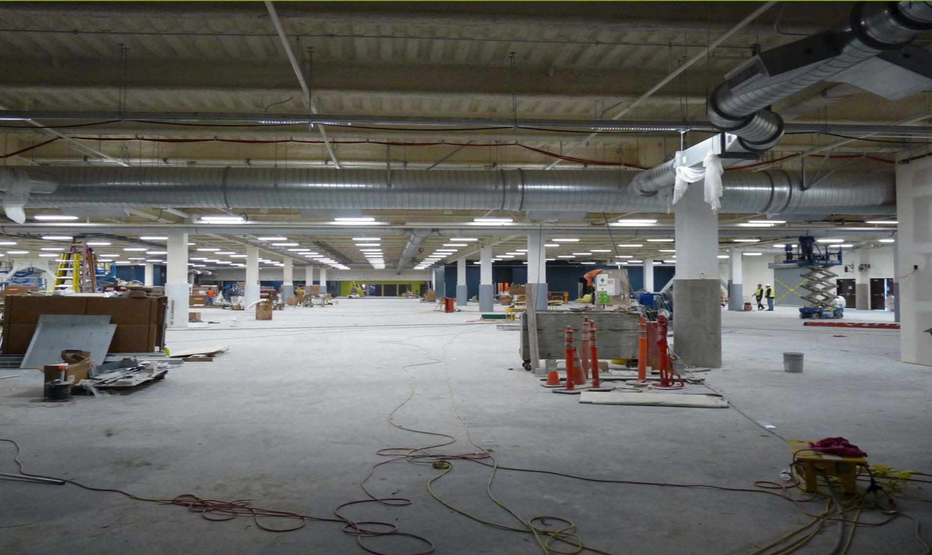
Ground Floor (Looking North)
