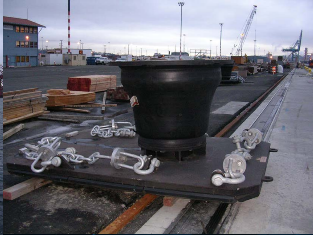
Terminal 30 Unit Fender Installation
