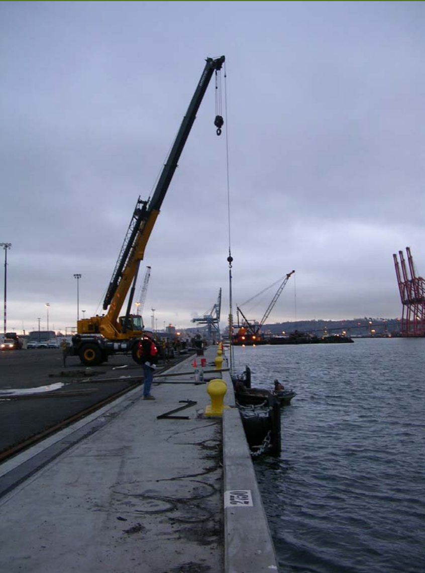
Terminal 30 Unit Fender Installation
